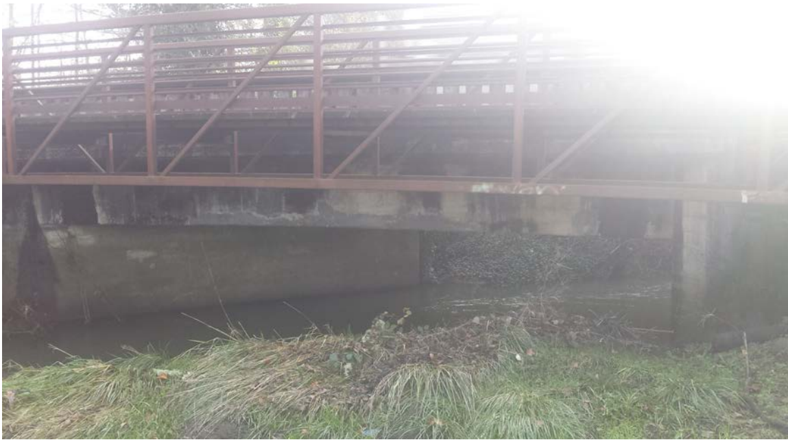
Figure 2. Cozine Creek Upstream Site showing Old Sheridan Road Bridge; photo 12/07/16.
